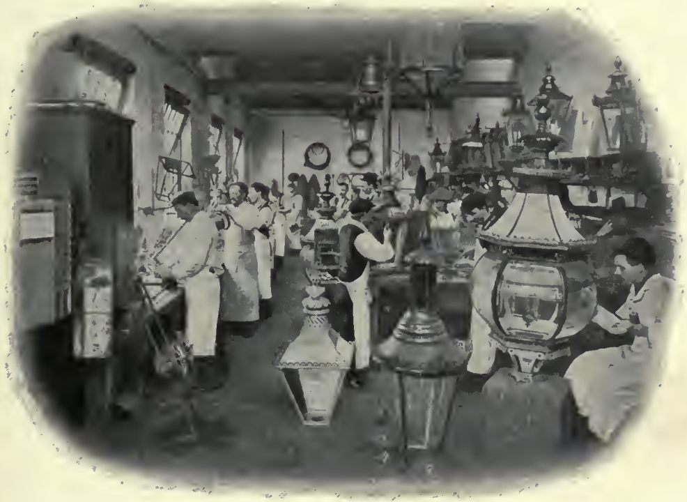
LAMP REPAIRING SHOP (SOUTH METROPOLITAN GAS COMPANY).
