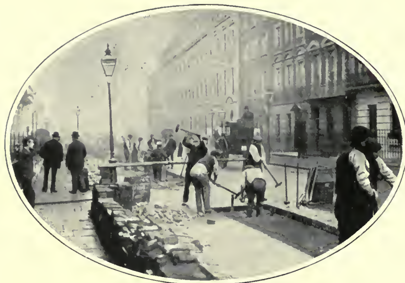
LAYING ELECTRIC CABLES.
